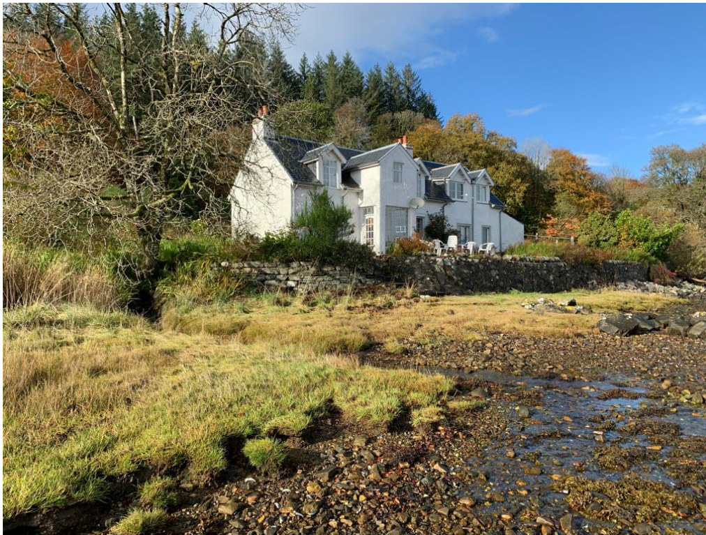
The Old Manse, Lochgair Shoreline – has a protruding elevation with broken eaves line, white harling, black slates, pitched roof dormers
